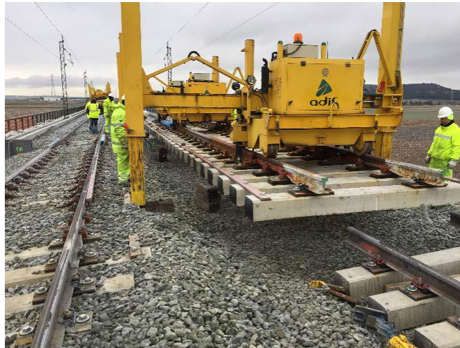
Plate 4.2 Rail panel handling machine
